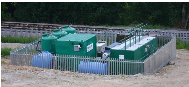
Figure 17.1.15-3 Example of a Groundwater Pump-and-Treat System
