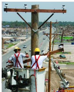
Figure 10.1.15-5: Crews Repair Poles After the May 22 Tornado
