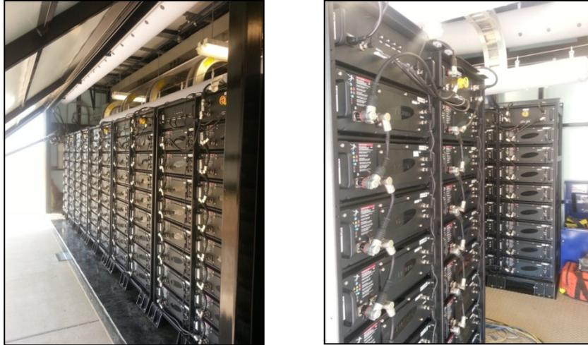
Figure 84. Racks of Batteries within the BESS Container
