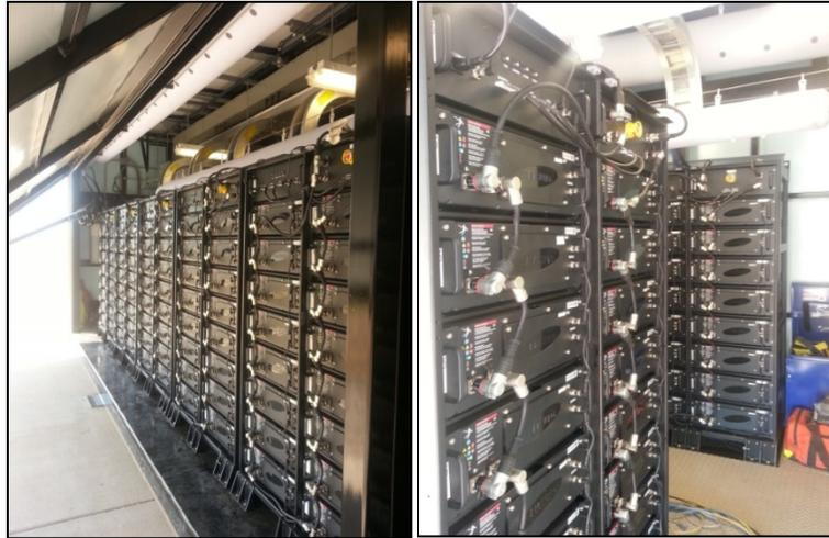
Figure 10. Racks of Batteries within the BESS Container
