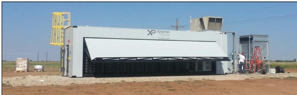
Figure 83. BESS Installed at the Reese Technology Center
