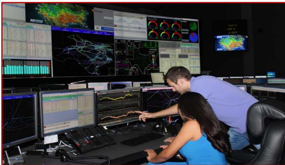
Figure 6. RTDMS Provides Grid Reliability Indicators at ERCOT
