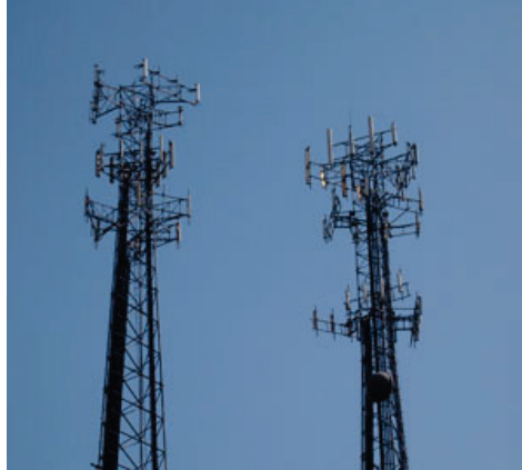
Figure 2.4.2-1: Lattice Cell Tower with Multiple Panel Antennas
