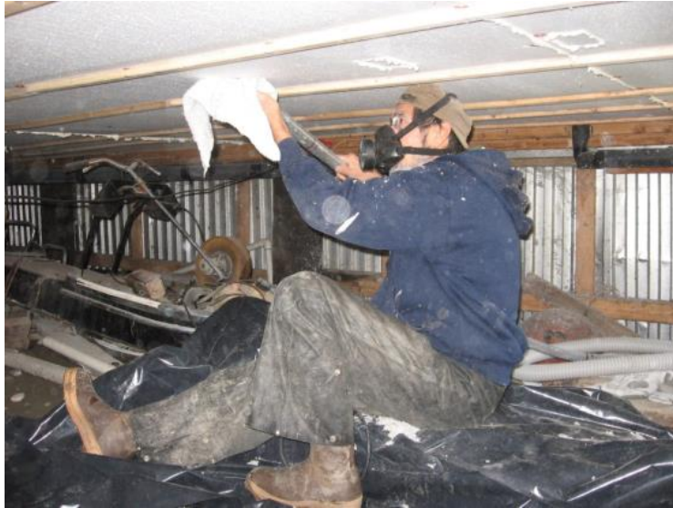
Dense-packing floors with cellulose
