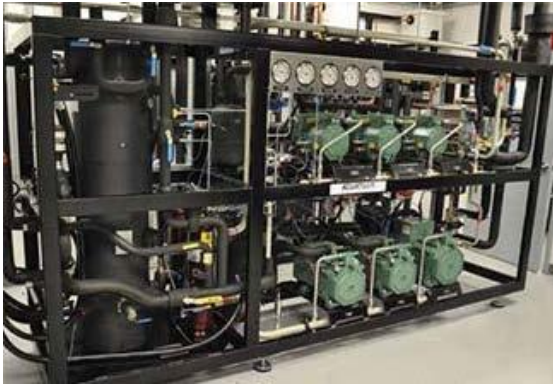
Hillphoenix's Parallel Rack System with Advansor™
