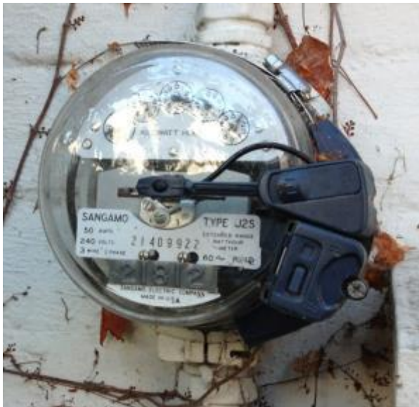
Utility approved Blueline device attached to utility meter.
