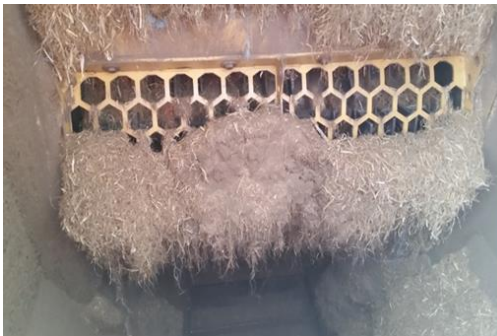
Plugging of hammer mill screen
