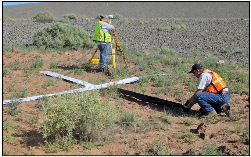
Surveyors install a ground control station for the Bluewater, New Mexico, Disposal Site LiDAR survey.
