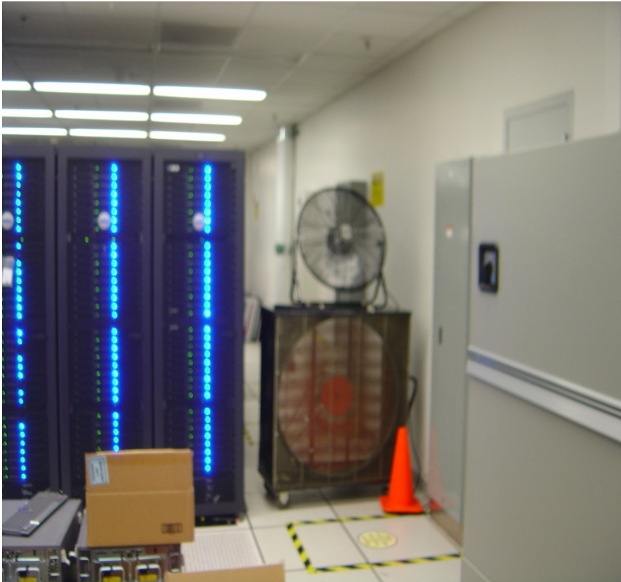
Fans were used to redirect air
