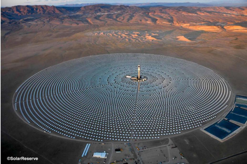
**Figure 5. 110-MW<sub>e</sub> Crescent Dunes Solar Energy Project in Tonopah, Nevada, with 10 hours of thermal storage. (source: SolarReserve)**
