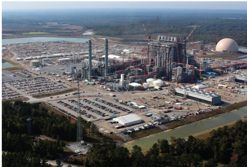
Southern Company Services, Inc. of Birmingham, Alabama, is developing an air-blown IGCC power plant large-scale demonstration project utilizing a coal-based transport gasifier. The project will deploy the Selexol physical solvent technology to demonstrate about 67% CO<sub>2</sub> removal, roughly three million tons per year. A sixty-mile CO<sub>2</sub> pipeline has been built to connect to an existing CO<sub>2</sub> pipeline used for enhanced oil recovery.
