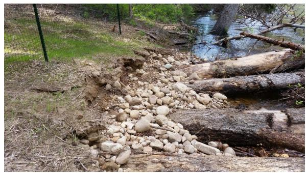
Figure 57: Example of previous in-stream wood placement along the Chewuch River. The bare soil was seeded and the riparian planting were on the other side of the mesh fencing. Rock armoring along the stream bank would help reduce erosion.
