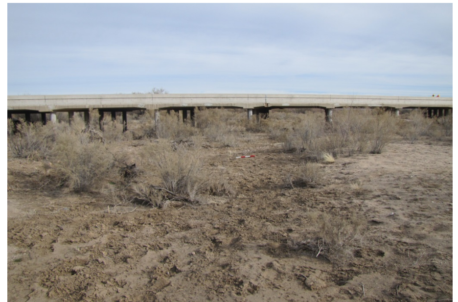
Gilson Wash, Photo 4. View downstream toward Gilson Wash Bridge from the high-flow area between the east and west channels, facing northeast.
