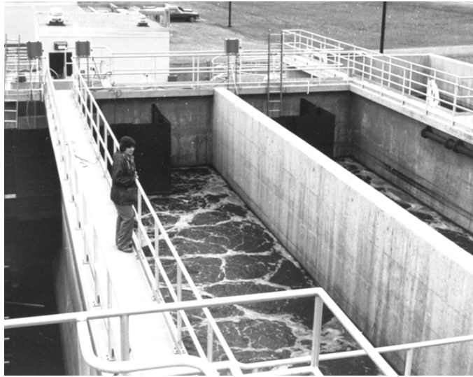
Figure 115. Activation of Four Large Aeration Tanks at the New X-6619 Sewage Treatment Plant (1983)
