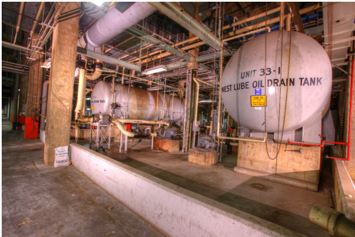
Figure 54. Unit X-33-1 Lube Oil Drain Tank (2010)
