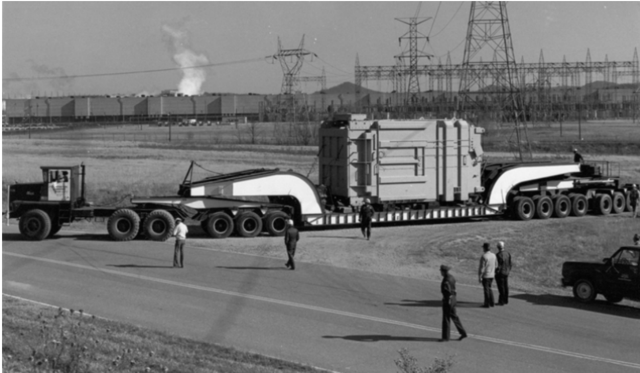
Figure 173. Transformer Being Installed in the Switchyards
