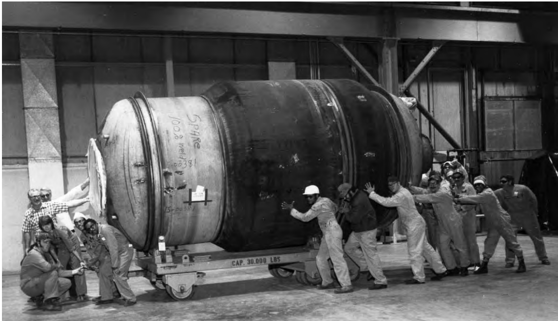
Figure 174. Converter Removed from the Cell for Retrofitting during CIP/CUP (1982)
