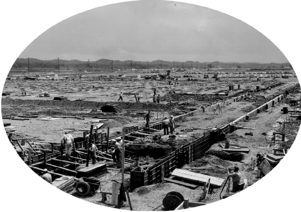
Figure 56. Construction underway for the X-330 Process Building Foundations (1953)
