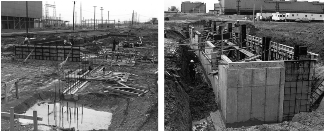
Figure 71. Construction of Foundations for the X-343 Feed, Vaporization, and Sampling Facility (1981)
