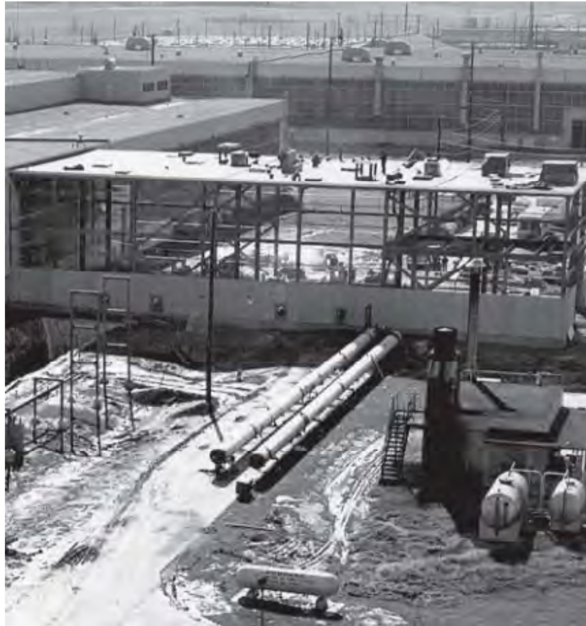
Figure 119. Construction of the West Side of the X-700 Converter Shop and Chemical Cleaning Facility to House the Furnace Stand (1955)
