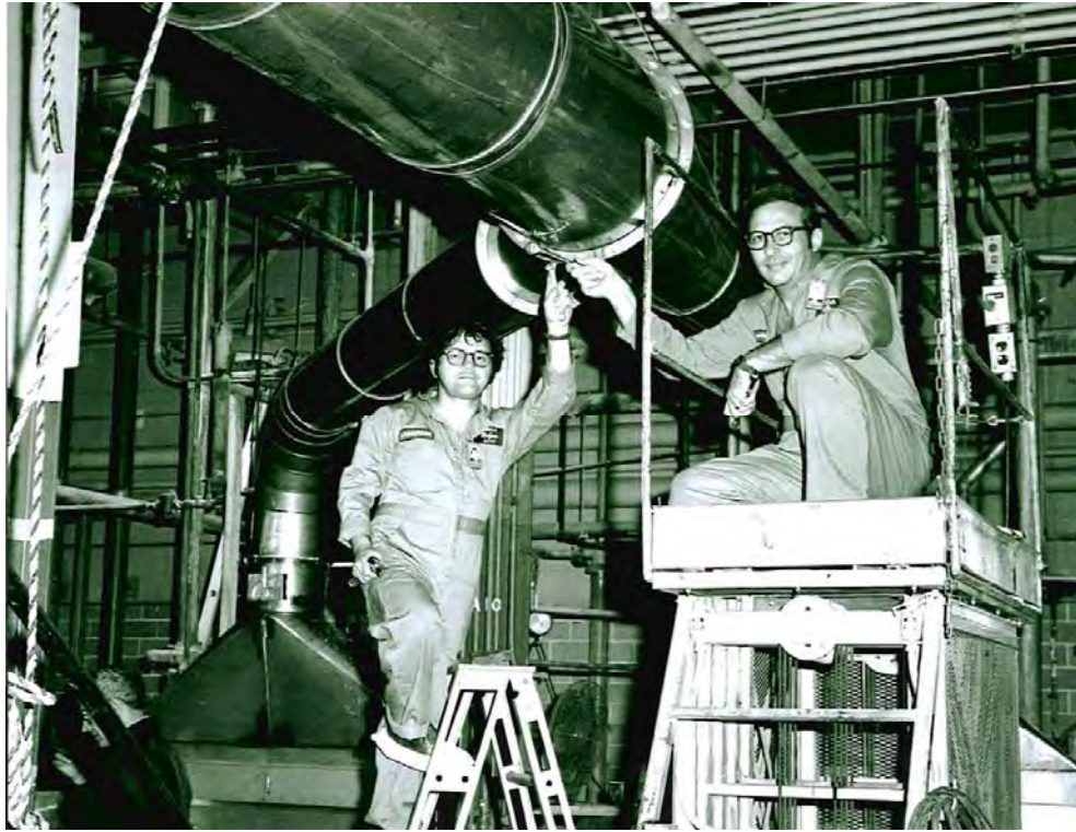
Figure 35. PORTS Workers Assembling Fabricated Piping (1954)
