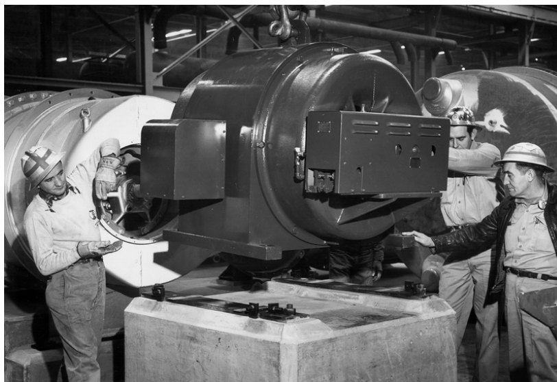
Figure 61. The First Compressor Motor Installed in the X-330 Process Building (1953)
