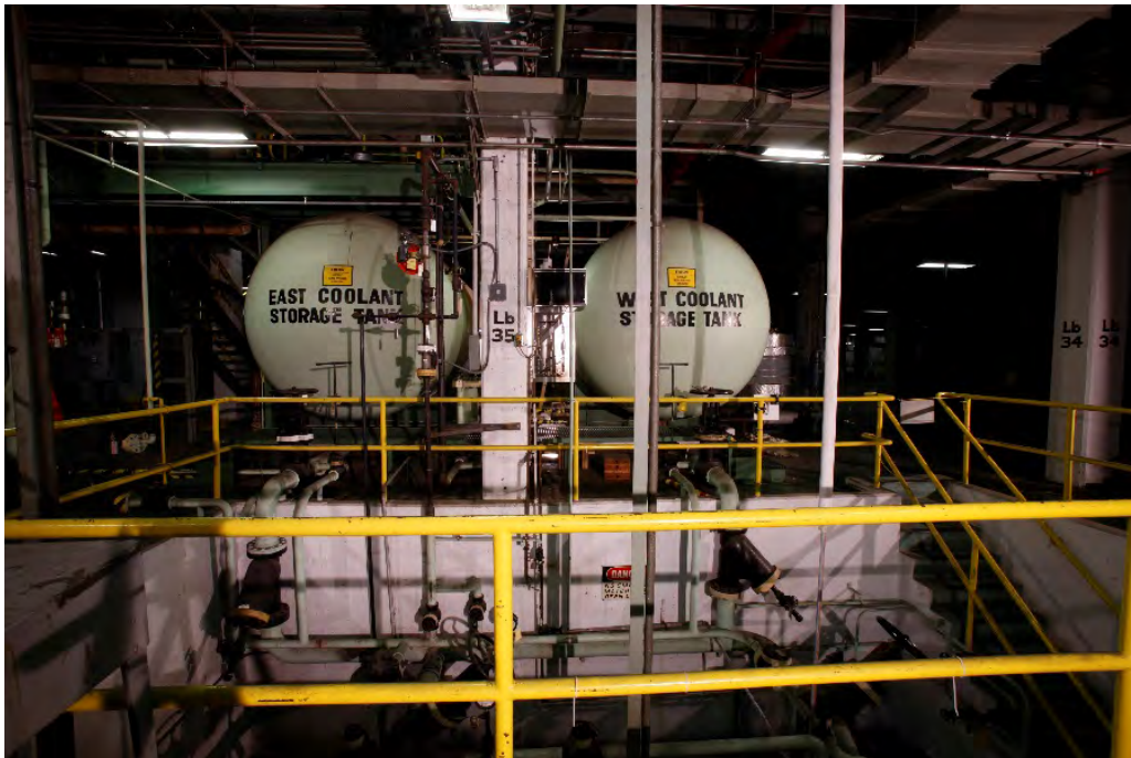
Figure 55. X-333 Process Building Coolant Storage Tanks (2010)
