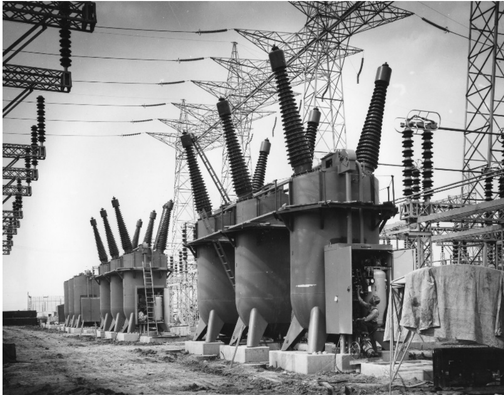
Figure 36. Large Oil Circuit Breakers in the Former X-533 Electrical Switchyard Complex (1954)
