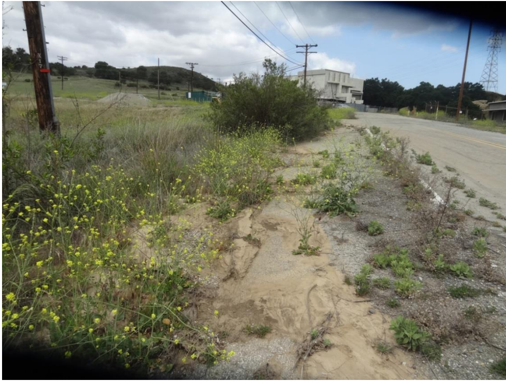
Photo 3 (May 7, 2014) above depicts a roadside drainage (15A on Figure I-5) created to drain runoff from developed upland areas, such as building pads; this drainage was identified in the survey as “non-waters of the U.S.” Photo 4 (May 7, 2014) below shows downstream, where this ephemeral drainage had left the roadside and clearly exhibited developed bed and banks; this drainage was identified as “waters of the U.S.” (15B in Figure I-5).
