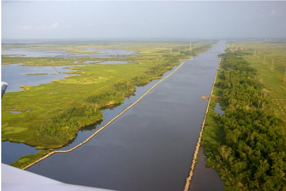
Exhibit 1 – Aerial View of GIWW near Valve Stations WH-4 and WH-5: south bank to the left. Source: Panoramio – Photos by stefkuna.
