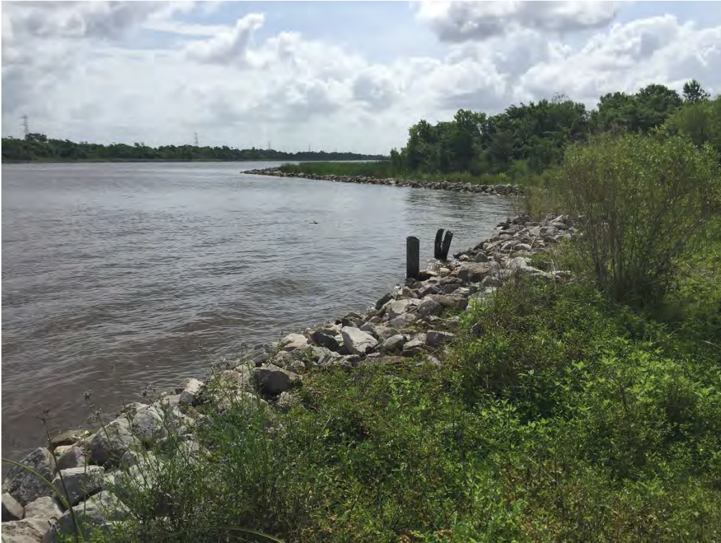
Photo 3 – WH-5 landing site with rip-rap stabilized bank.
