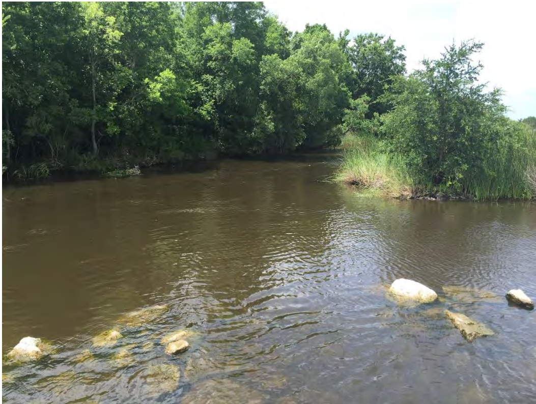
Photo 2 – View of WH-4 spoil bank looking south into Vinton Drainage Canal and showing rip-rap barrier to access.
