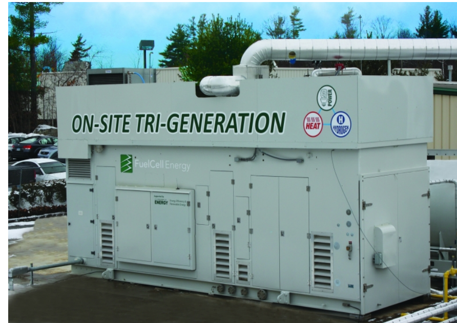
The high efficiency packaged CHHP system in operation at FuelCell Energy's manufacturing plant in CT .
