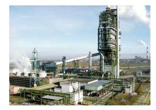
LEFT: MIDREX<sup>™</sup> DRI shaft furnaces are being installed around the world to use various reducing gases and solids
