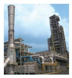
BELOW: The ZR Process accepts any reducing gas source – direct natural gas, syngas from a coal gasifier, coke oven gas or  $H_2/CO$  mixtures.
