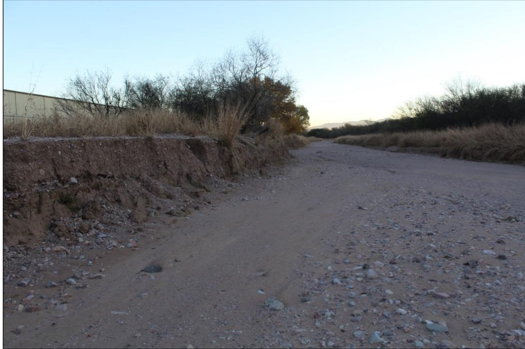
Looking east at Mariposa Canyon Wash in section 5 of the Project area
