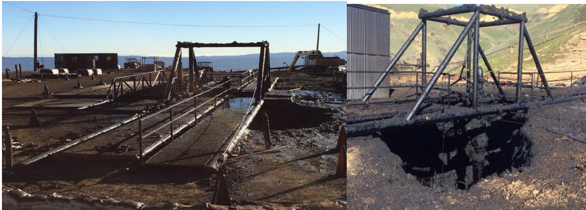
Figure 10: Vent crater caused by expulsion of top kill attempt materials.
