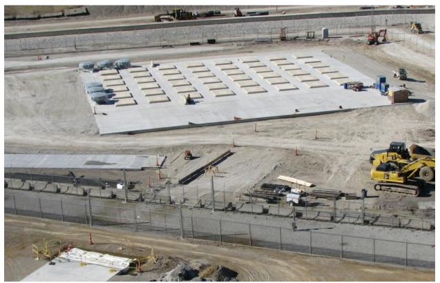
Figure A3-6 Holtec HI-STORM UMAX, Completed Pad Construction, Callaway ISFSI
