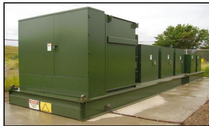
Modular Integrated Transportable Substation (MITS)
