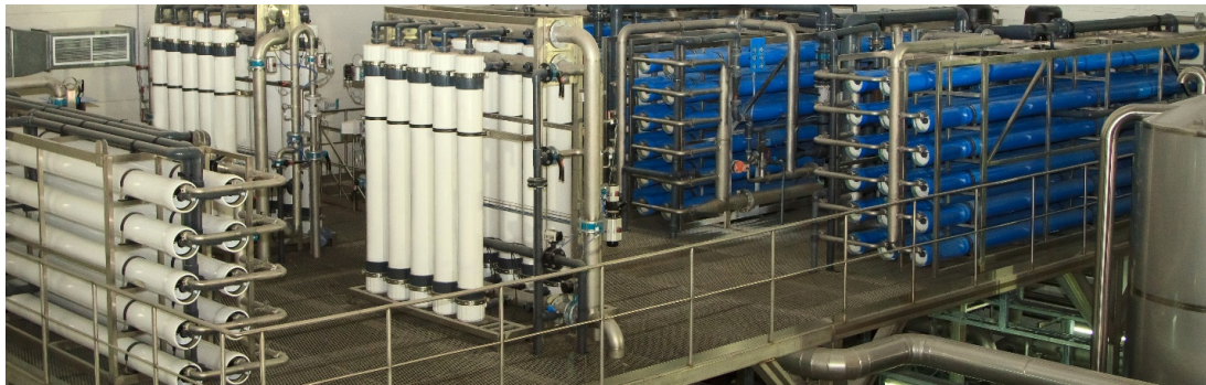
Figure 2 - The Claude "Bud" Lewis Carlsbad Desalination Plant near San Diego removes salt from 50 million gallons of seawater every day and is a prime example of implementing existing technology to find new sources of water in the arid West.
