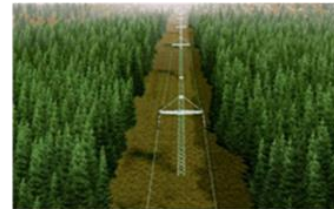
One \pm 500kV DC bipole
