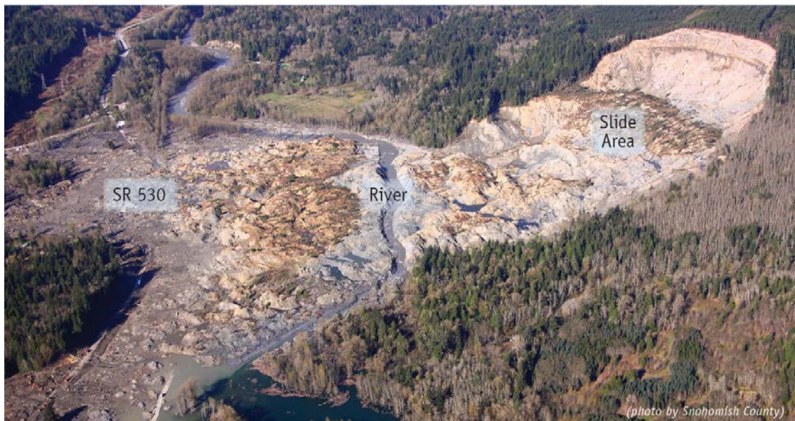
Figure 8.1.15-5: Aerial View of the Oso Landslide and Damage to SR 530
