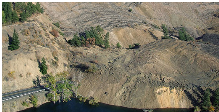
Photo of the 2009 Nile Landslide
