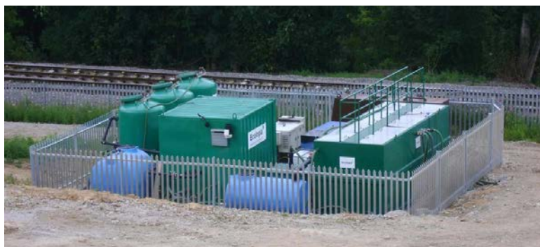
Figure 17.1.15-3 Example of a Groundwater Pump-and-Treat System
