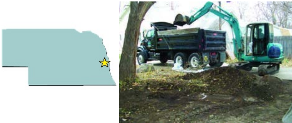
Figure 12.1.15-3: Track Hoe Excavating Contaminated Surface Soil
