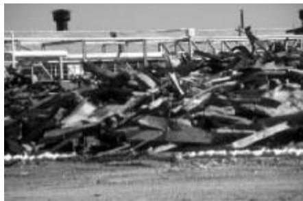
Low-level radioactive scrap metal from a building demolition at uranium processing facility
