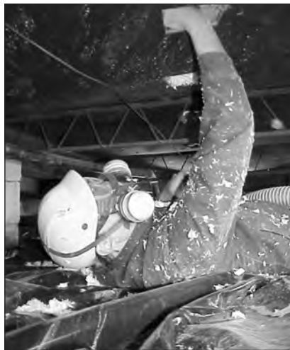
After cutting access holes through the belly board of the mobile home, push any existing insulation aside so that the flexible fill tube can slide the length of the joist cavity for a complete fill.
