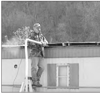
A worker blows fiberglass into the cavity of the mobile home roof. Note the 2 x 4s used as wedges to hold the roof cavity open. A small amount of blowback can be seen.
