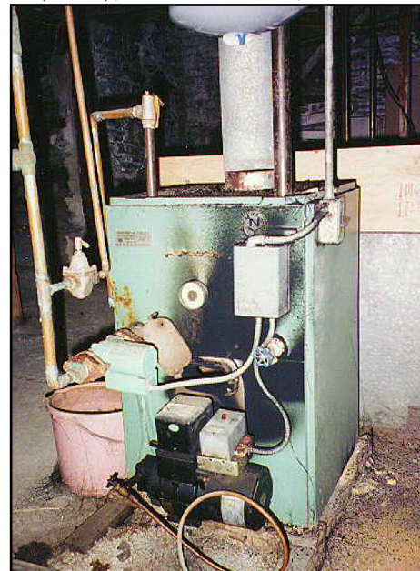
Obvious evidence of drafting failure
