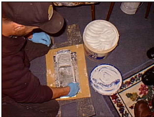
Sealing a register boot with duct mastic
