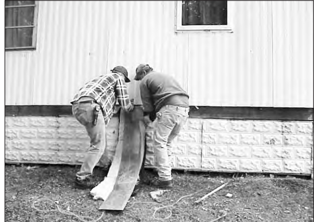
(left) To fill the outer area of the mobile home floor, a muffler pipe is attached to the flexible hose. The natural curve of the pipe makes it easy to rotate the pipe in the cavity to get maximum fill. (right) Batt stuffing is one way to reinsulate the walls of mobile homes. Remove the bottom two rows of screws, and you can stuff the insulation into the cavity using a strong, flexible plastic stuffer.
