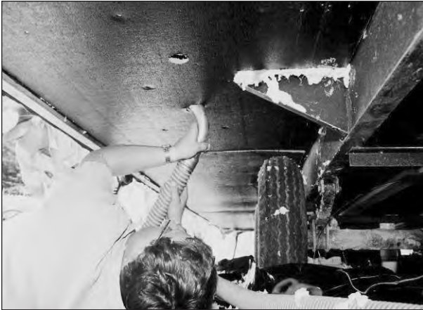
(left) To fill the outer area of the mobile home floor, a muffler pipe is attached to the flexible hose. The natural curve of the pipe makes it easy to rotate the pipe in the cavity to get maximum fill. (right) Batt stuffing is one way to reinsulate the walls of mobile homes. Remove the bottom two rows of screws, and you can stuff the insulation into the cavity using a strong, flexible plastic stuffer.
