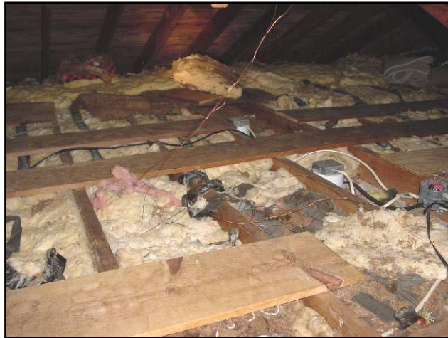
Some attics require much preparation work before they can be blown with cellulose
