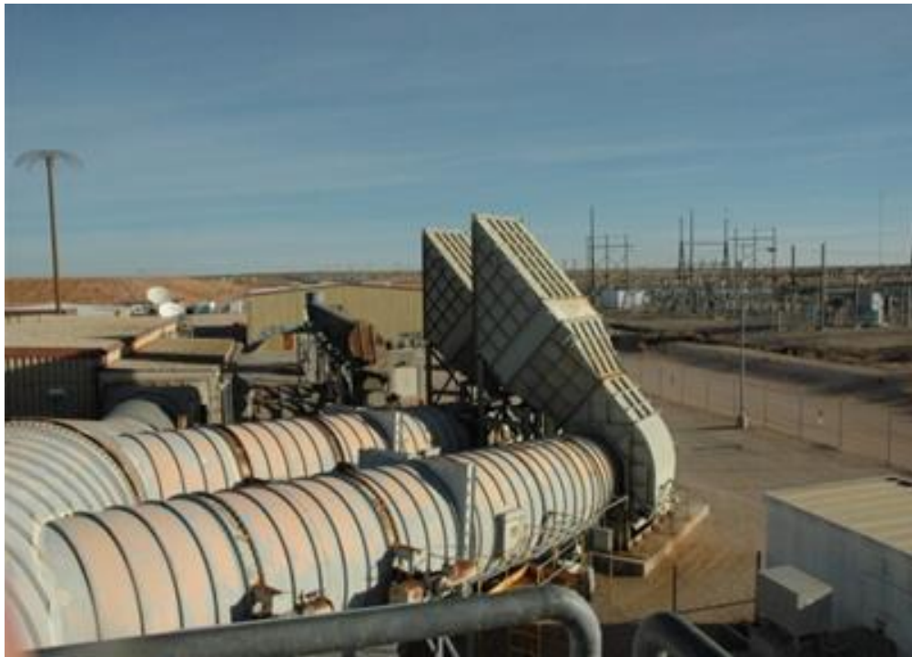
Figure 19: Ventilation Fans 700A and 700B
