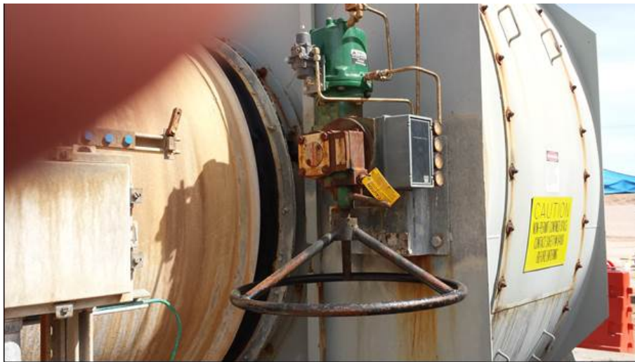
Figure 11: 860 Vortex Manual Hand Wheel
