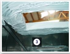
A properly fastened and sealed boot to duct connection: This prop represents a type of duct configuration commonly seen in mobile homes.
