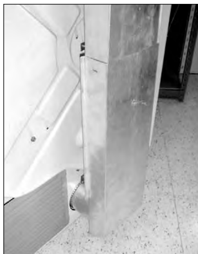
(left) If space is tight between the dryer and the wall, a periscope vent allows the dryer to be 2 inches closer to the wall. (right) I stuck this gauge's right-angled terminal tube into a vertical section of the vent to measure static pressure.
