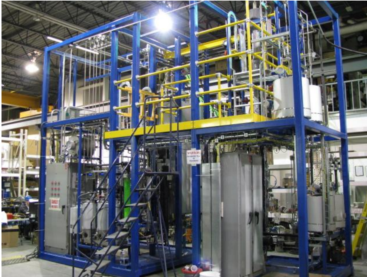
A view of the fixed bed reactor and distillation column used to make stabilized oils
