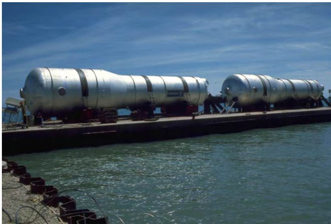
Figure 2-137. Steam Generators Being Delivered to Zion Site by Barge during Construction
