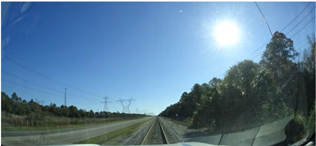
Figure 2-156. Onsite Industrial Rail Spur Approaching U.S. Highway 19 from the West (2015)
