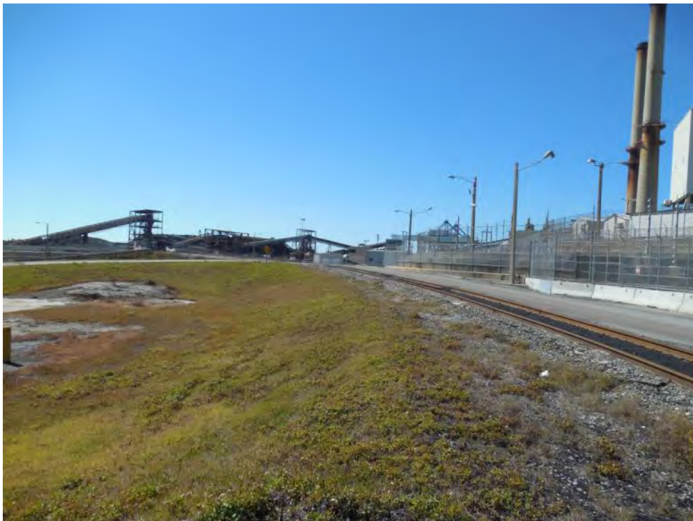
Figure 2-154. Onsite Industrial Rail Spur in Front of Future Independent Spent Fuel Storage Installation Site (Facing West) (2015)
