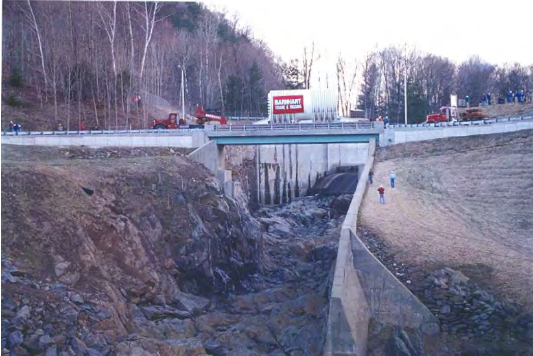
Photo courtesy of AREVA
