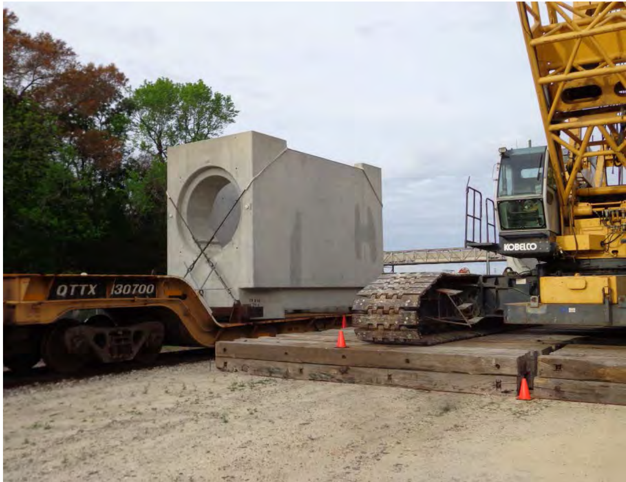
Figure 2-179. Horizontal Storage Module Staged for Unloading (2015)
