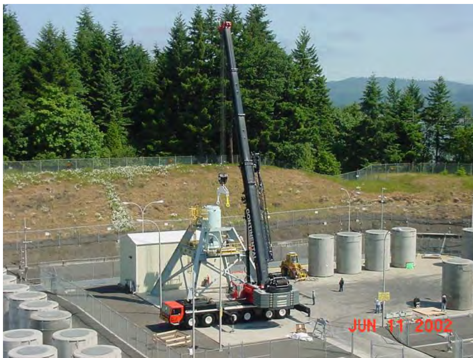
Photo courtesy of Trojan
