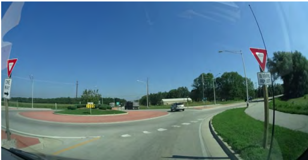
Figure 2-228. Traffic Circle on WI-310 (Looking East) (2014)
