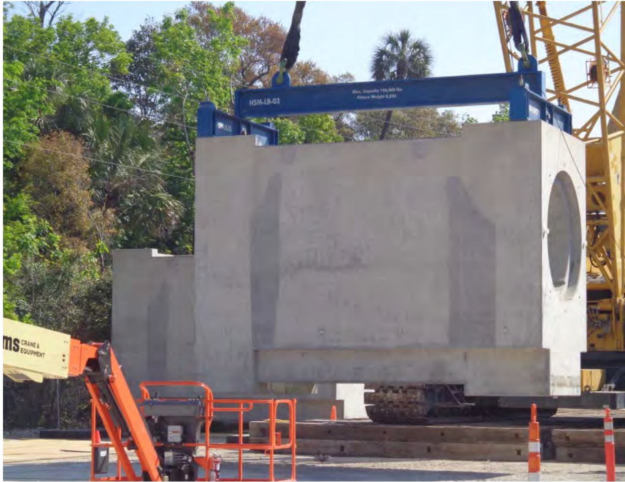
Figure 2-180. Horizontal Storage Module Being Unloaded from Railcar (2015)
