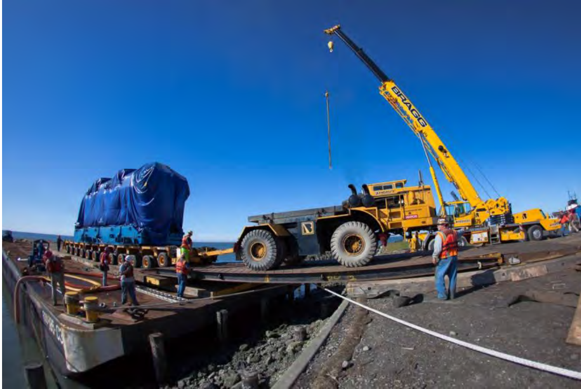
Photo courtesy of Bragg Crane & Rigging Co.
