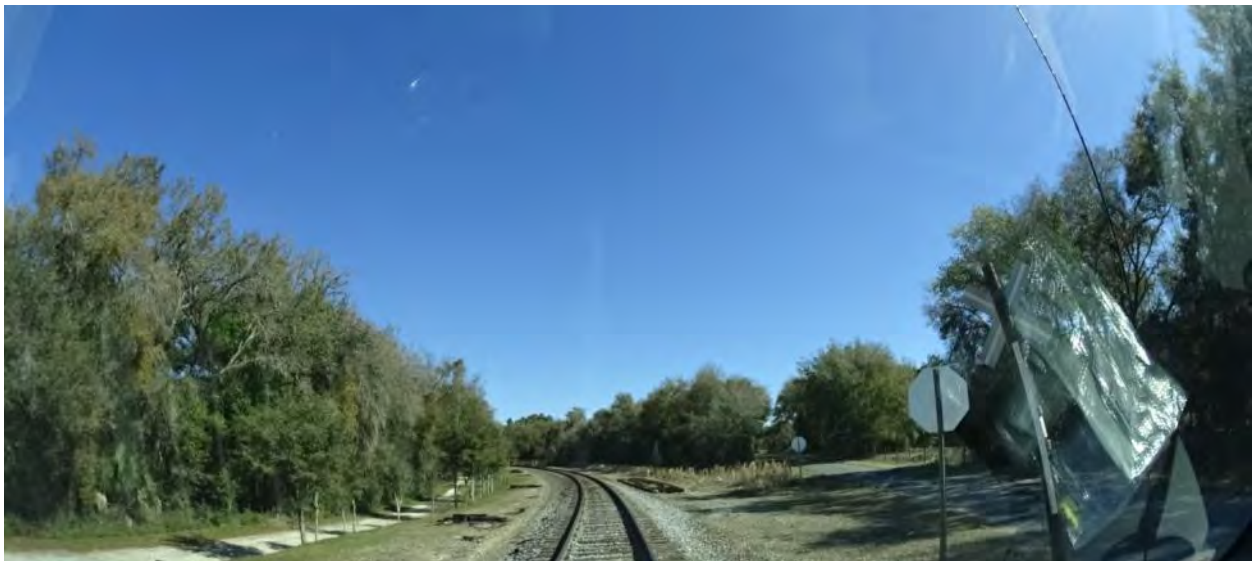
Figure 2-163. Florida Northern Railroad near Dunnellon, Florida (2015)
