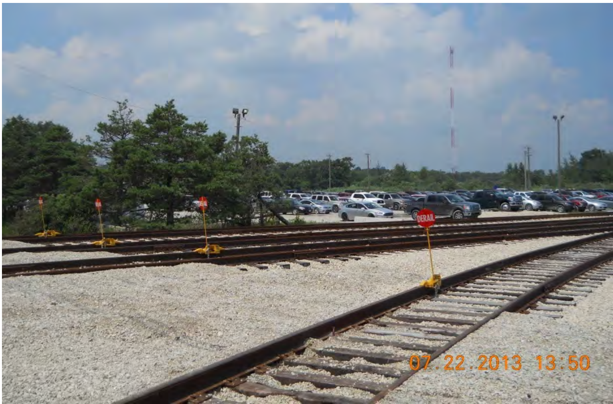
Figure B-20. Derailers Outside of Zion Site (2013)
