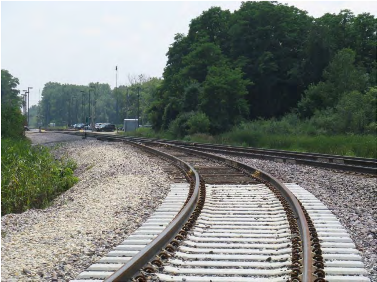
Figure 2-142. Junction of Zion On-site Rail Spur with Union Pacific Railroad Showing Concrete Rail Ties (2013)
