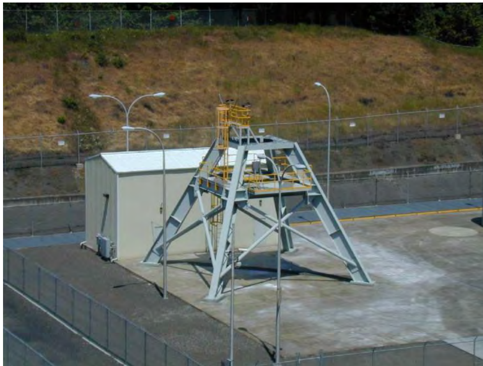
Photo courtesy of Trojan
