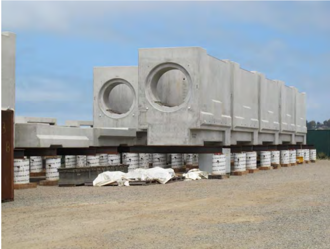
Figure 2-259. Horizontal Storage Modules (2015)
