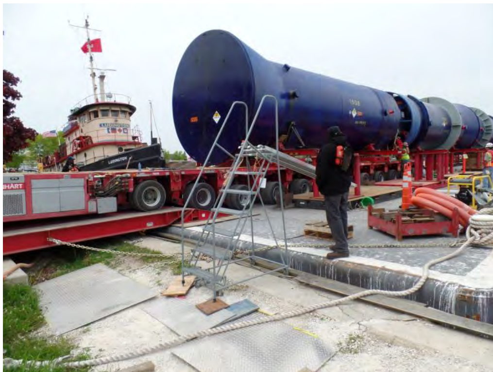
Figure 2-248. Fourth Steam Generator Moving onto Barge (2014)
