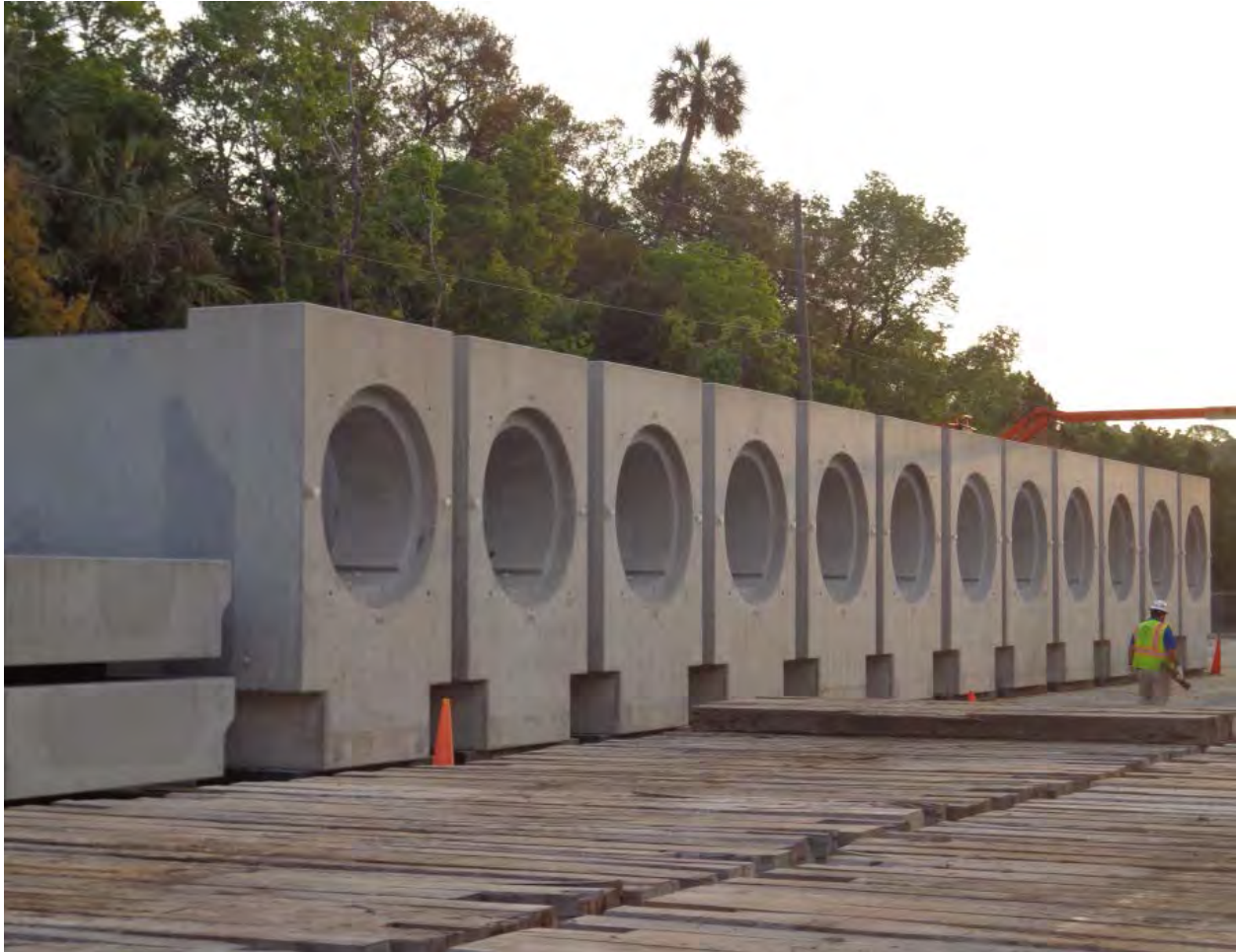
Figure 2-181. Horizontal Storage Modules at Nuclear Spur after Unloading (2015)
