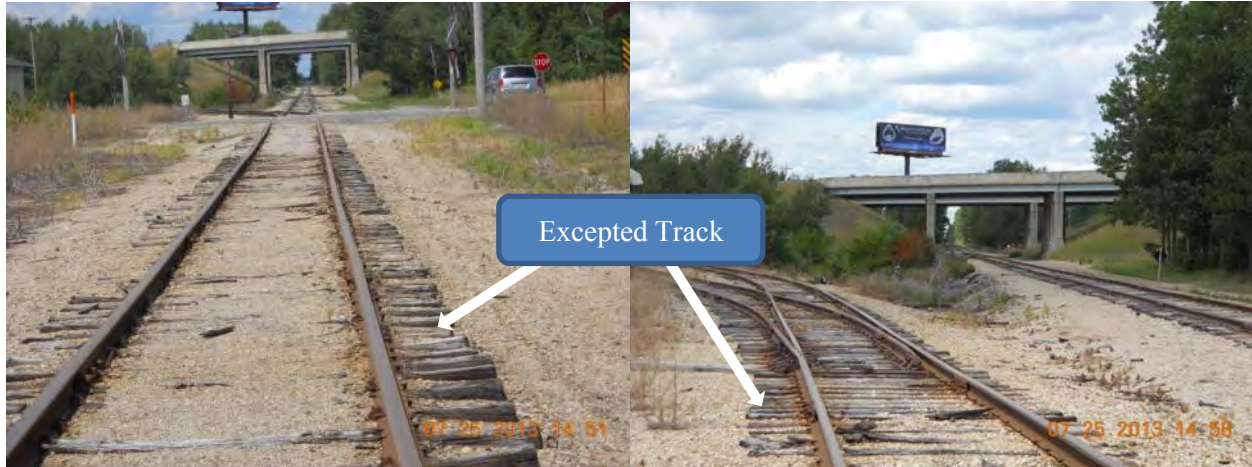
Figure B-8. Track Condition in the Vicinity of Gaylord Transload Location (Looking North) (2013)
