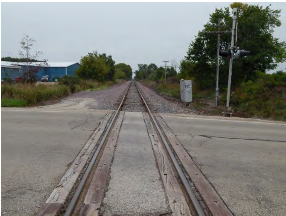
Figure 2-219. Potential Denmark Transload Location (Looking North) (2014)
