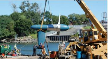
Verdant Power installs a testing device in the East River of New York City on August 29, 2012. Testing took 2 weeks and looked at new rotors and composite blades.
