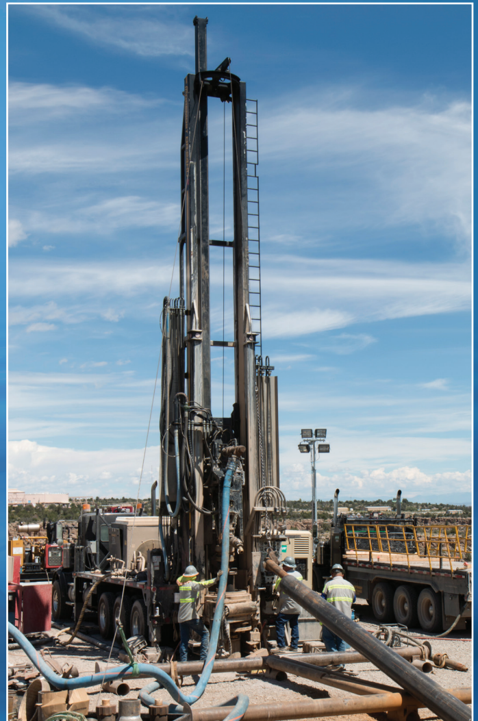
Drilling of a corehole in Mortandad Canyon.
