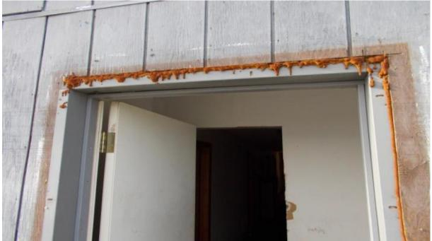
Figure 2. This was one of the older doors on the lodge, insulated around the frame but still with numerous air leaks around the entire frame and UV rays are reducing the effectiveness of the insulation
