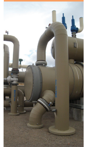
Geothermal piping, Steamboat Springs, NV
