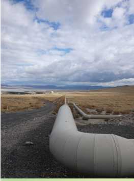
Geothermal piping, Fallon, NV
