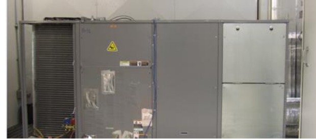
CCCHP system as installed in Psychrometric chamber at UTRC
