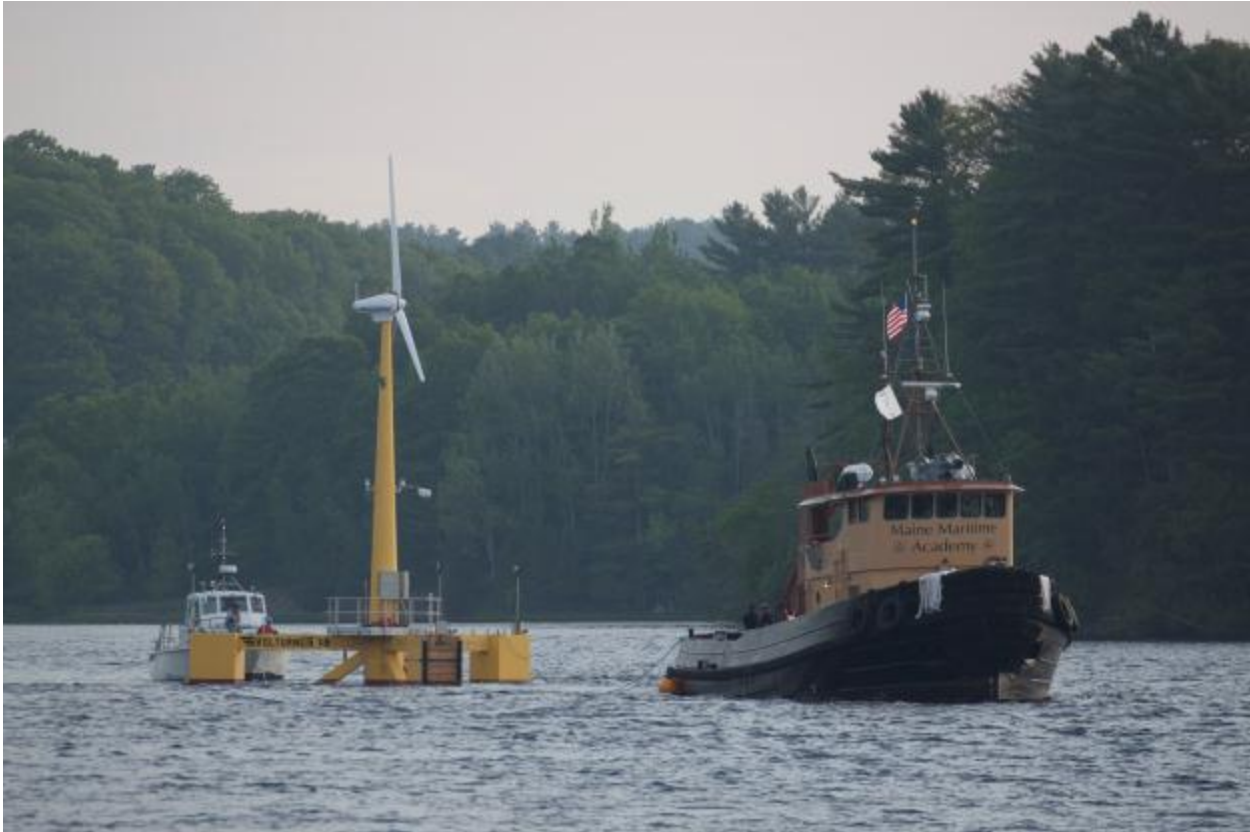
Figure 1 - The VolturnUS 1/8th-scale floating offshore wind turbine, being towed to the Castine site.
