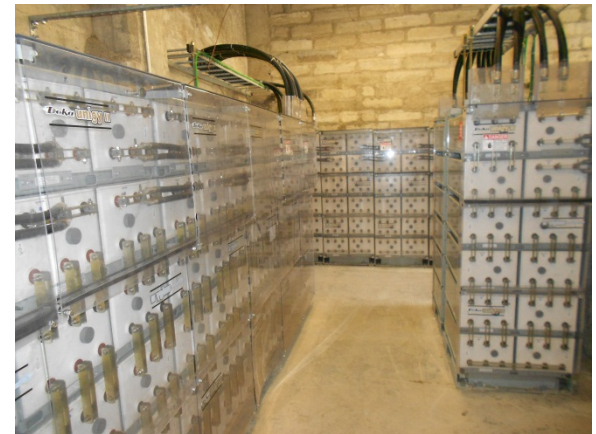
NPS Alcatraz PV system – a 307 kW PV Array, 2000 ah battery, inverter array and diesel system that can operate diesel off
