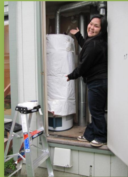
Installing water heater blankets and teaching maintenance
