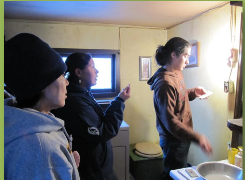
Insulating outlets and switches
