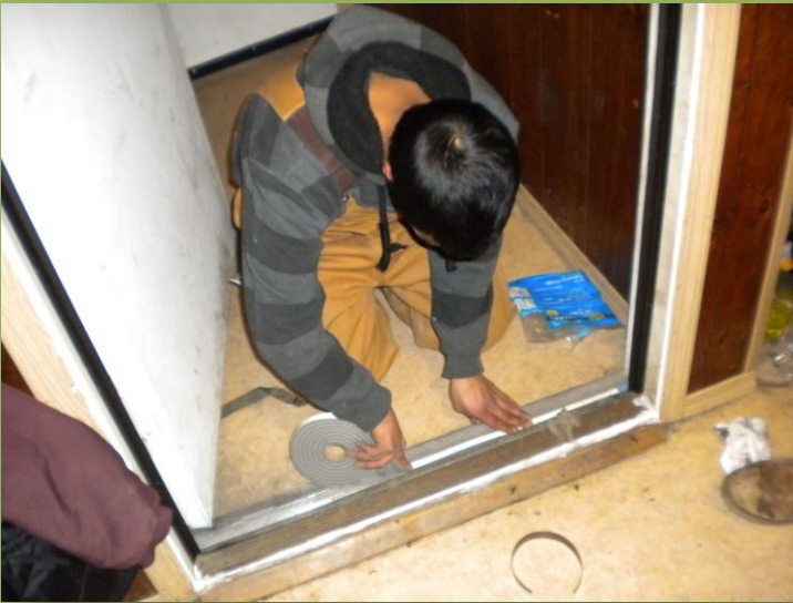
Installing door sweep and weather-stripping
