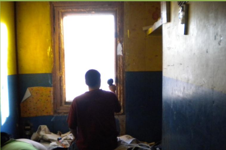
Applying window film
