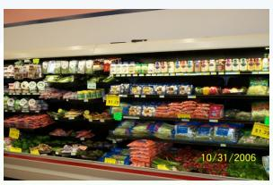
One project consists of purchasing and installing door freezers, produce cases, beverage coolers, and florescent light fixtures to replace the old, inefficient equipment. The technology in the replacement units will provide 41.9% energy savings.
