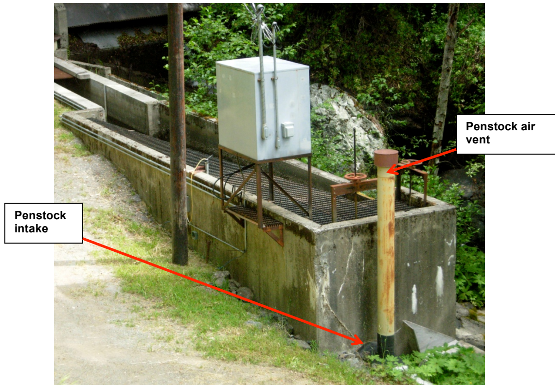
Figure 44: Bluford diversion channel for Zenia hydroelectric project
