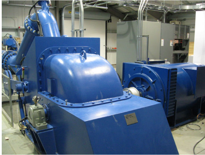
Figure 52: Twin-nozzle Pelton turbine and generator for a 1.1-MW hydroelectric plant in British Columbia, Canada
