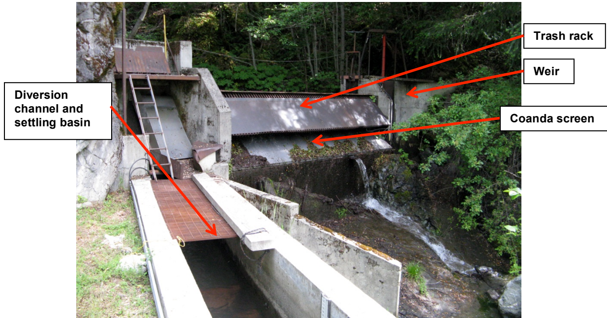
Figure 43: Bluford intake system for Zenia hydroelectric project
