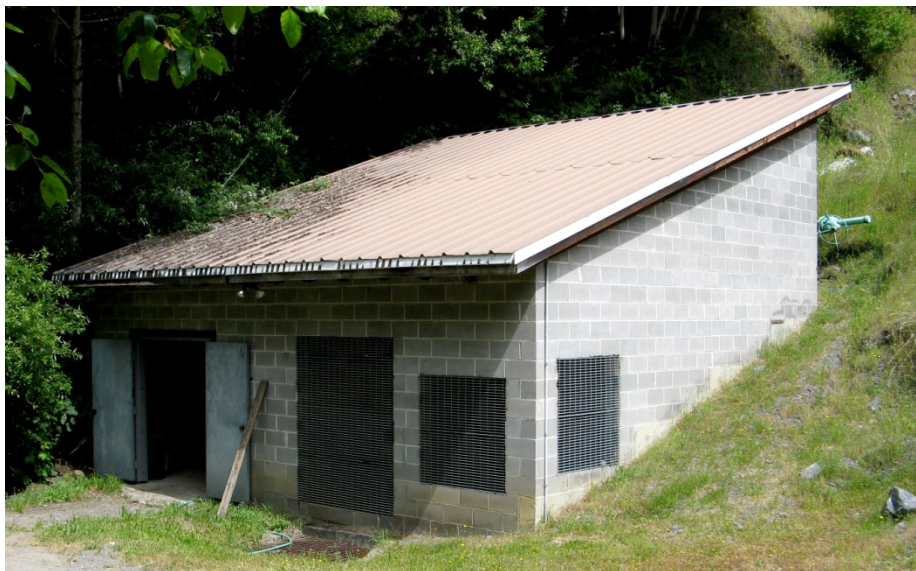
Figure 49: Powerhouse (27' x 27') for a 1.7-MW hydropower system in Zenia, CA
