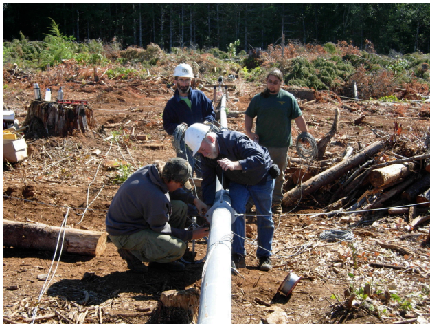
Installing sensors on the MET tower.
