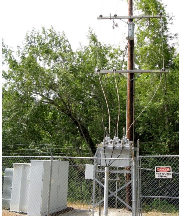
Figure 53: Small substation for a 1.7-MW hydropower system in Zenia, CA
