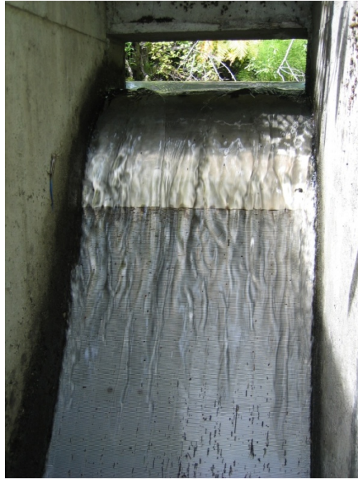
Figure 45: Self-cleaning Coanda-effect screen on intake system, Zenia hydroelectric project
