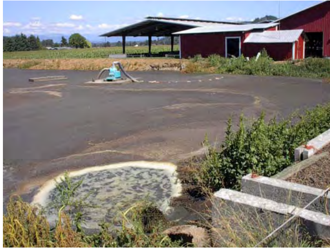
Storage pond receives separated liquid.
