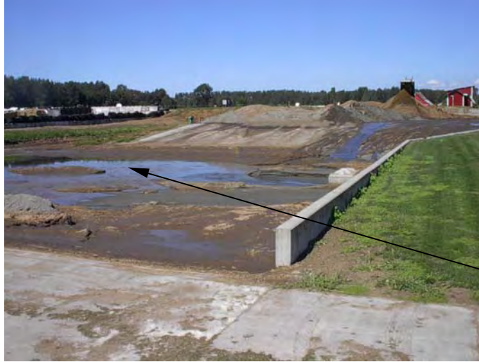
Pipe under the grass flows from gutter to sand settling pond
