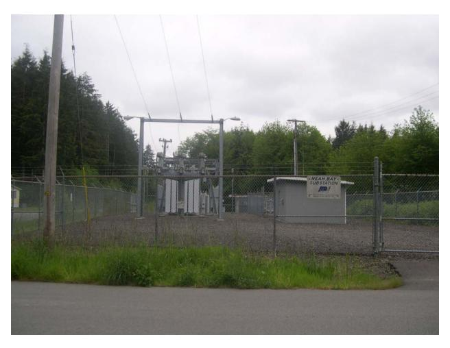
The substation is located on the corner of Young Doctor and Back Track road. There are three circuits identified as "A", "B", and "C" that extend from the substation and provide electric service to the town and region.
