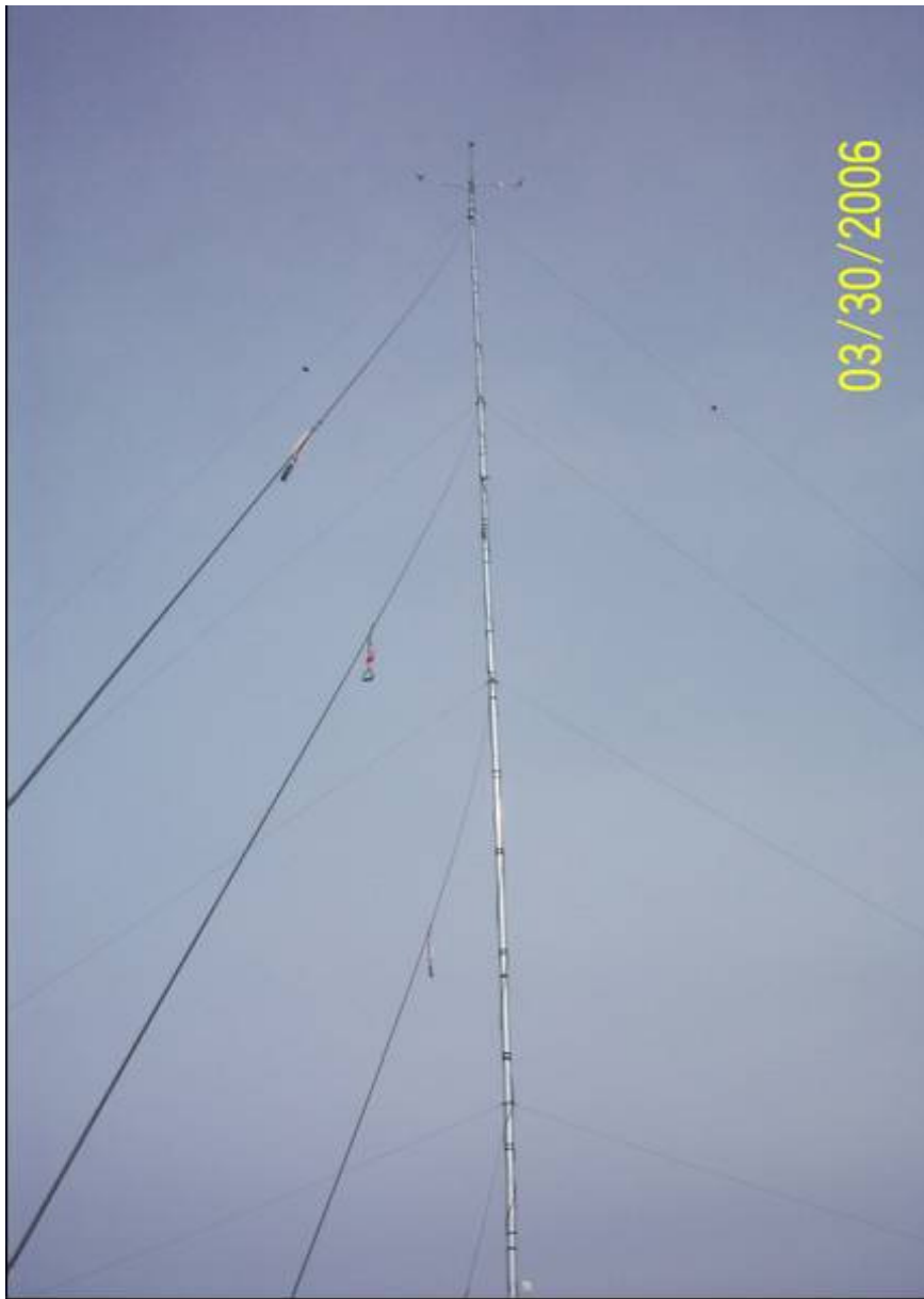
Photo 2: This is the wind monitoring tower loaned by Alaska Energy Authority to KIT to measure wind energy production potential. Note the bird deterrent devices hanging from the guy wires that were used to minimize bird collisions. The temperature sensor is the small device at the very bottom of the picture just to the right of the tower.
