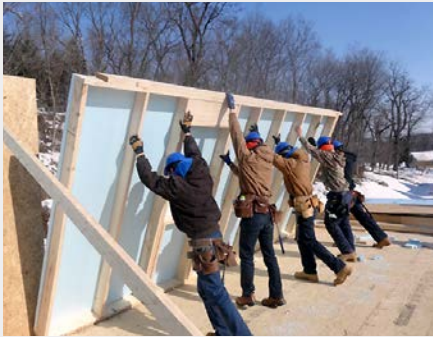
Typical wall section installation
