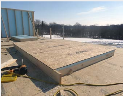
Sheathing over foam wall assembly
