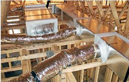
The insulated ducts were installed close to the ceiling and were well sealed.
