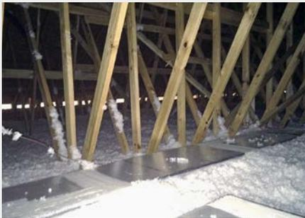
After attic insulation was installed (shown), additional R-30 insulation was mounded above the ducts.
